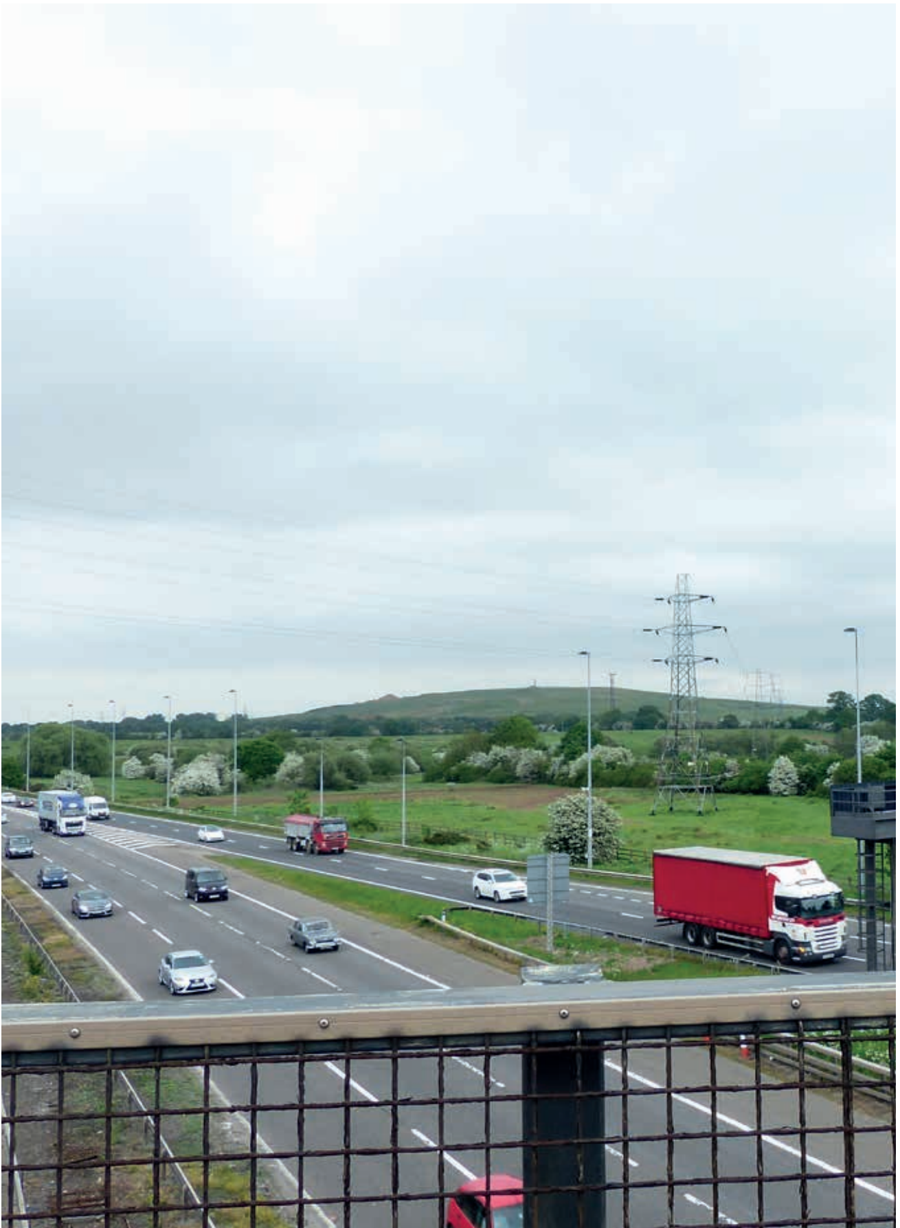
FIGURE 10: M42 AND UTILITIES CORRIDOR BETWEEN THE NEC AND ARDEN CROSS, IMAGE, ARUP
