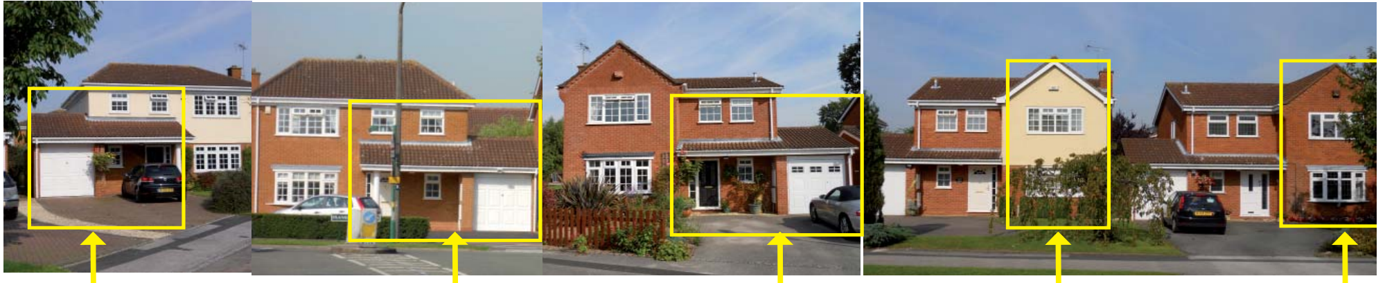
The pitched roof extends over the garage and provides a porch to the main entrance to the house. The porch roof is often supported by a column/pillar which is a distinct feature of housing built at this time. The basic proportions of the houses types are similar, there is however some variation in the use of materials.
