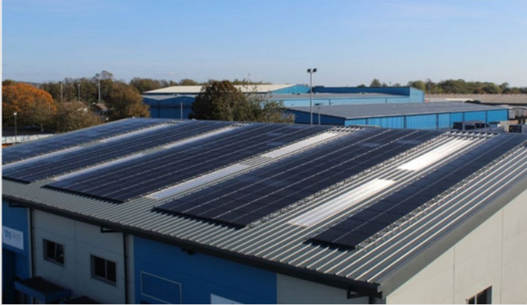
Figure 11: Image of the solar installation on Portsmouth City Council industrial units. 1
