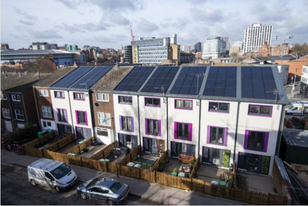
Figure 8: Image of Energiesprong retrofit of housing in Nottingham. 1
