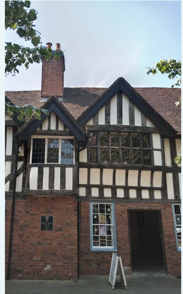
The Manor House 126 High Street
