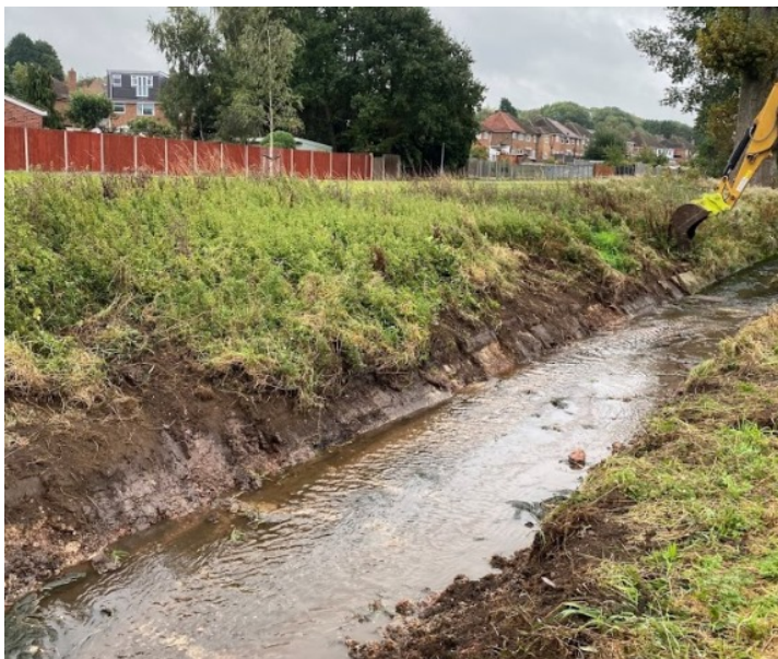
Excavation of the existing brook prior to re-profiling
