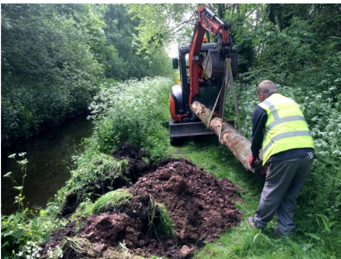
Installing timber at Low Brook, 2018
