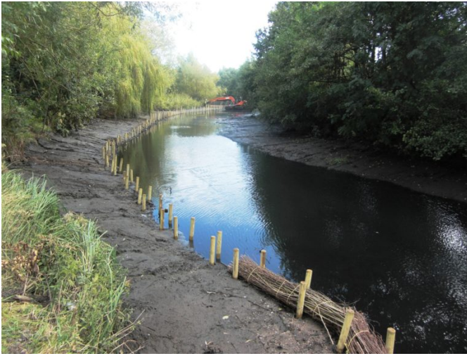
Brushwood bank reinforcement, October 2019
