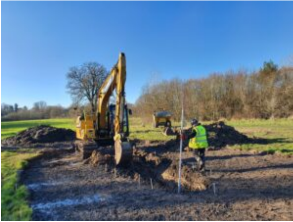
Excavating the pond in January 2022.
