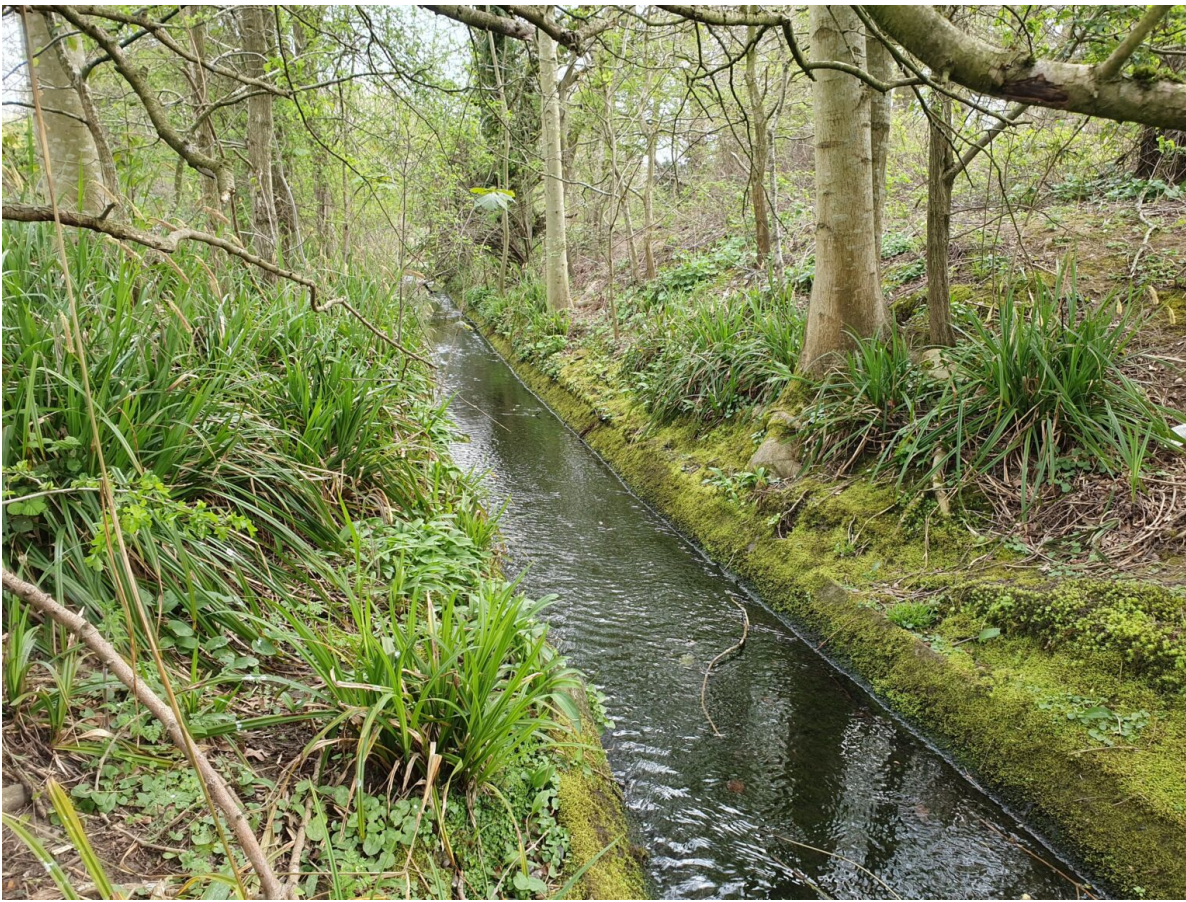
Concrete lined Alder Brook (upstream of the pond) prior to restoration
