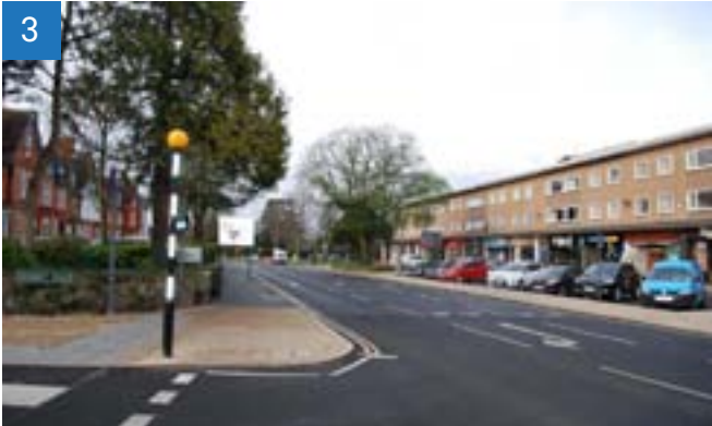
3 Station Road looking west towards Blossomfield Road Roundabout: Has recently undergone improvements as part of the Solihull Gateway Project, including upgraded public realm and improved pedestrian priority.
