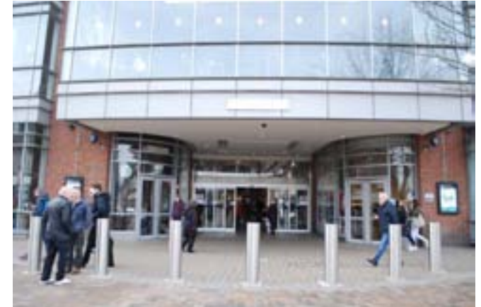
Entrance of Touchwood Shopping Centre
