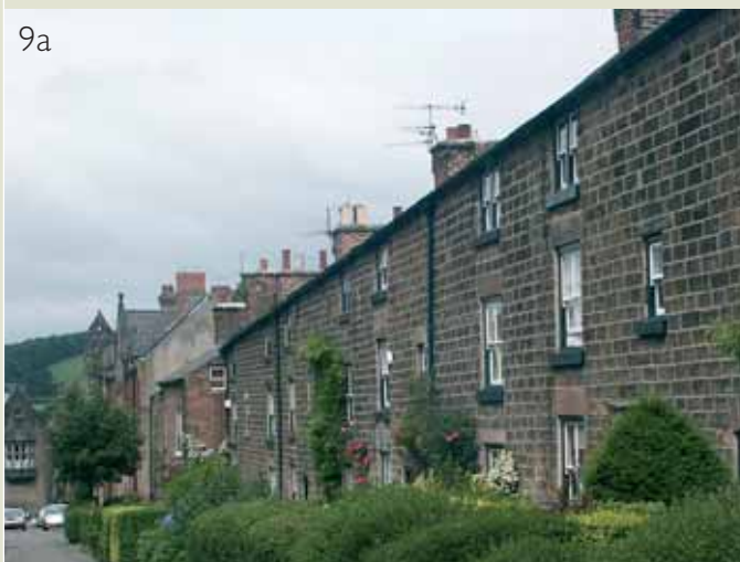
9b Strutt Estate, Belper: 2-storey millworkers' houses, Long Row © The Paul Drury Partnership
