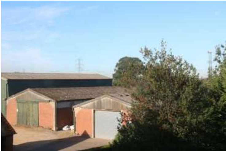
Figure 16 Park Farmhouse, view from first floor west to barns
