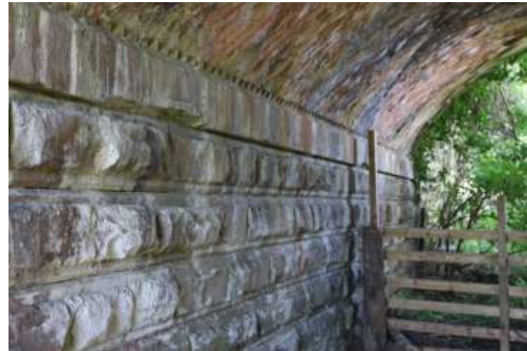
Figure 24 Railway bridge over west drive showing rusticated rock faced stone with dog-tooth dentil detail along top course
