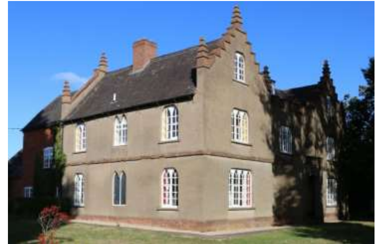
Figure 14 Park Farmhouse, east elevation facing Packington Park
