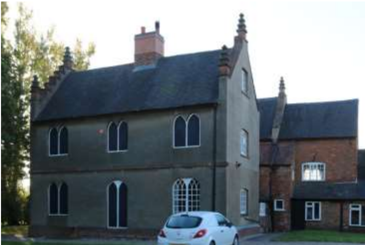
Figure 13 Park Farmhouse, north elevation
