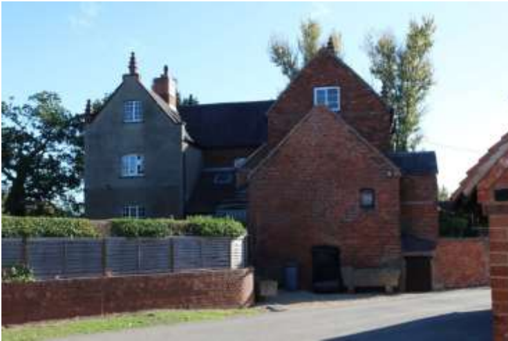
Figure 12 Park Farmhouse, west elevation
