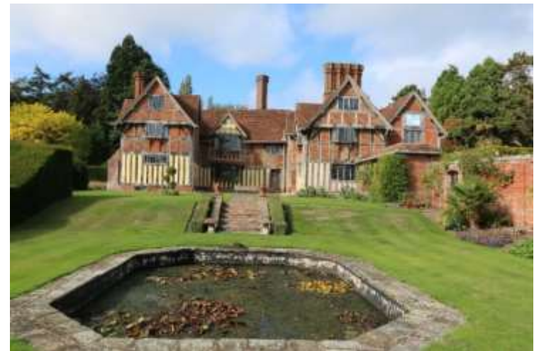
Figure 12 Grimshaw Hall; east rear elevation
