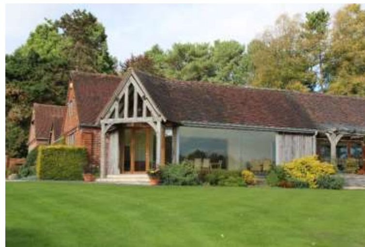
Figure 14 Converted and extended farm buildings north of hall
