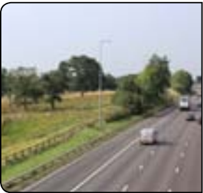
Photograph 2.2: The M42 motorway segregates this area into two parts.
