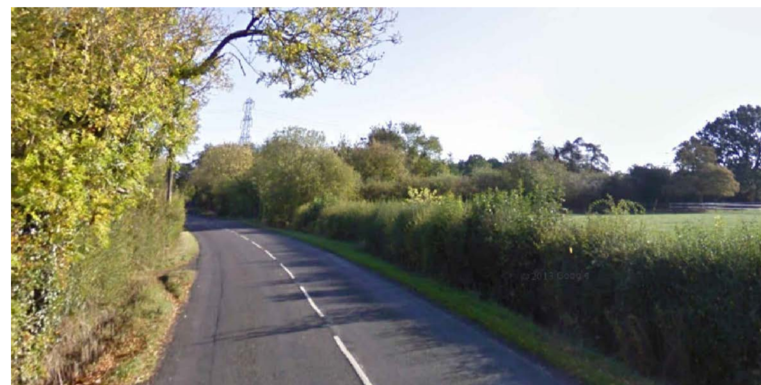
View along Waste Lane looking Eastbound
