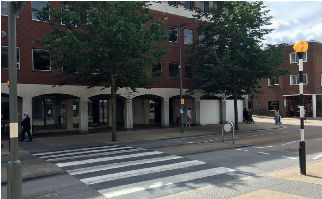
→ Photograph of Solihull Gateway
