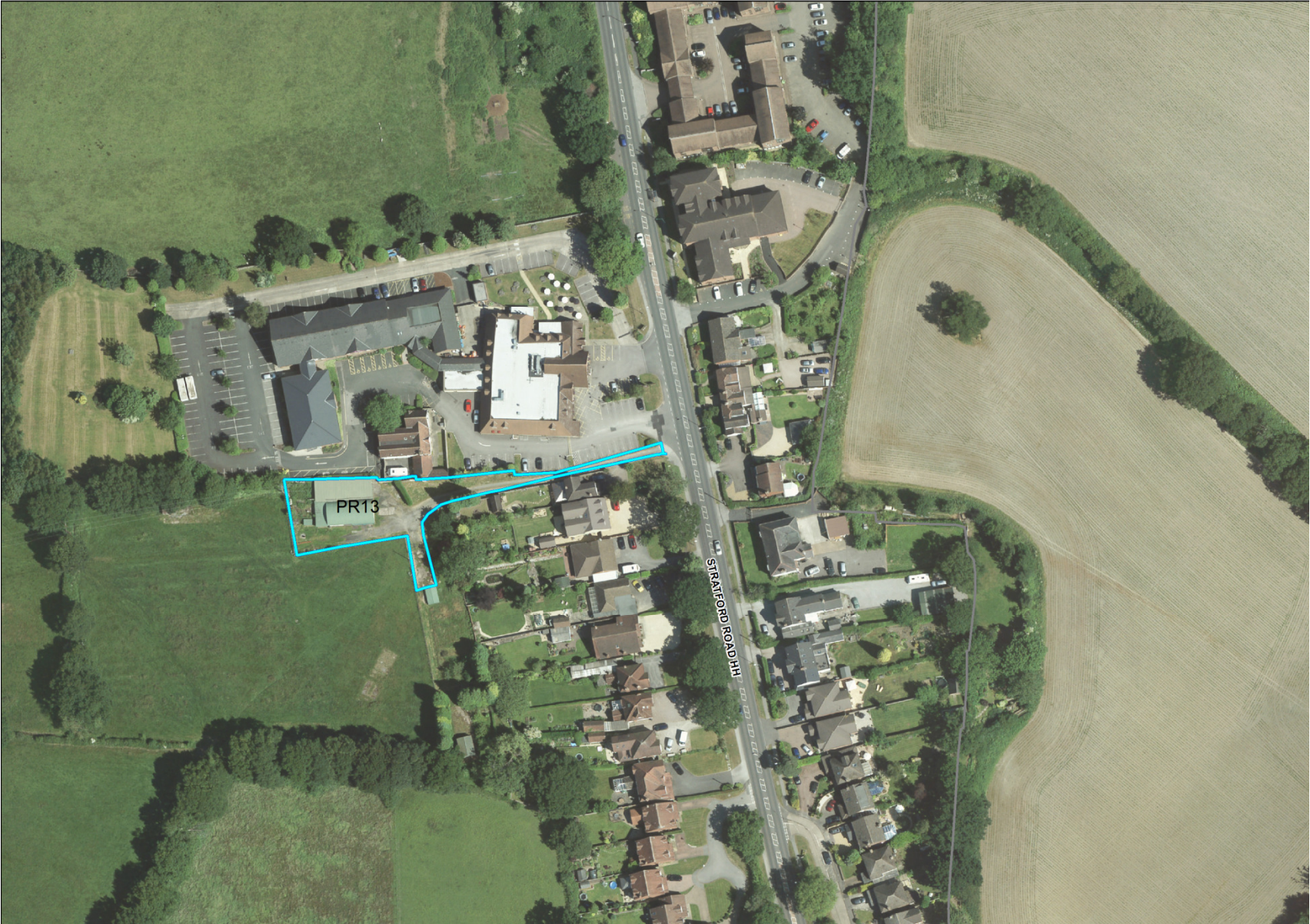
PR13 - Workshop, 2180 Stratford Road
