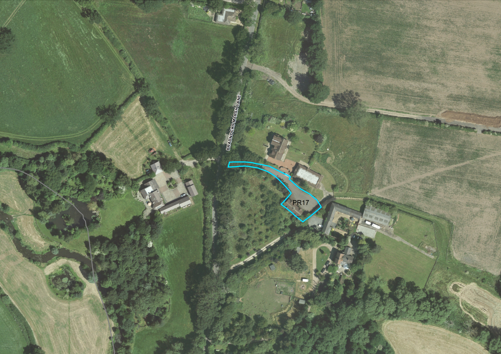
PR17 - Garage Oakfield Farm, Bradnocks Marsh Lane
