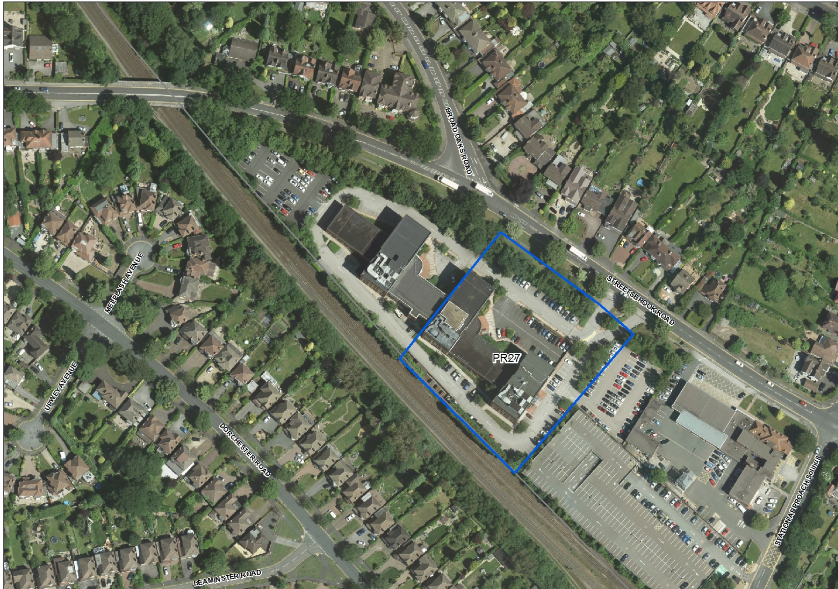
PR27 - Sapphire House (East), Streetsbrook Road, Solihull B91 1RD
