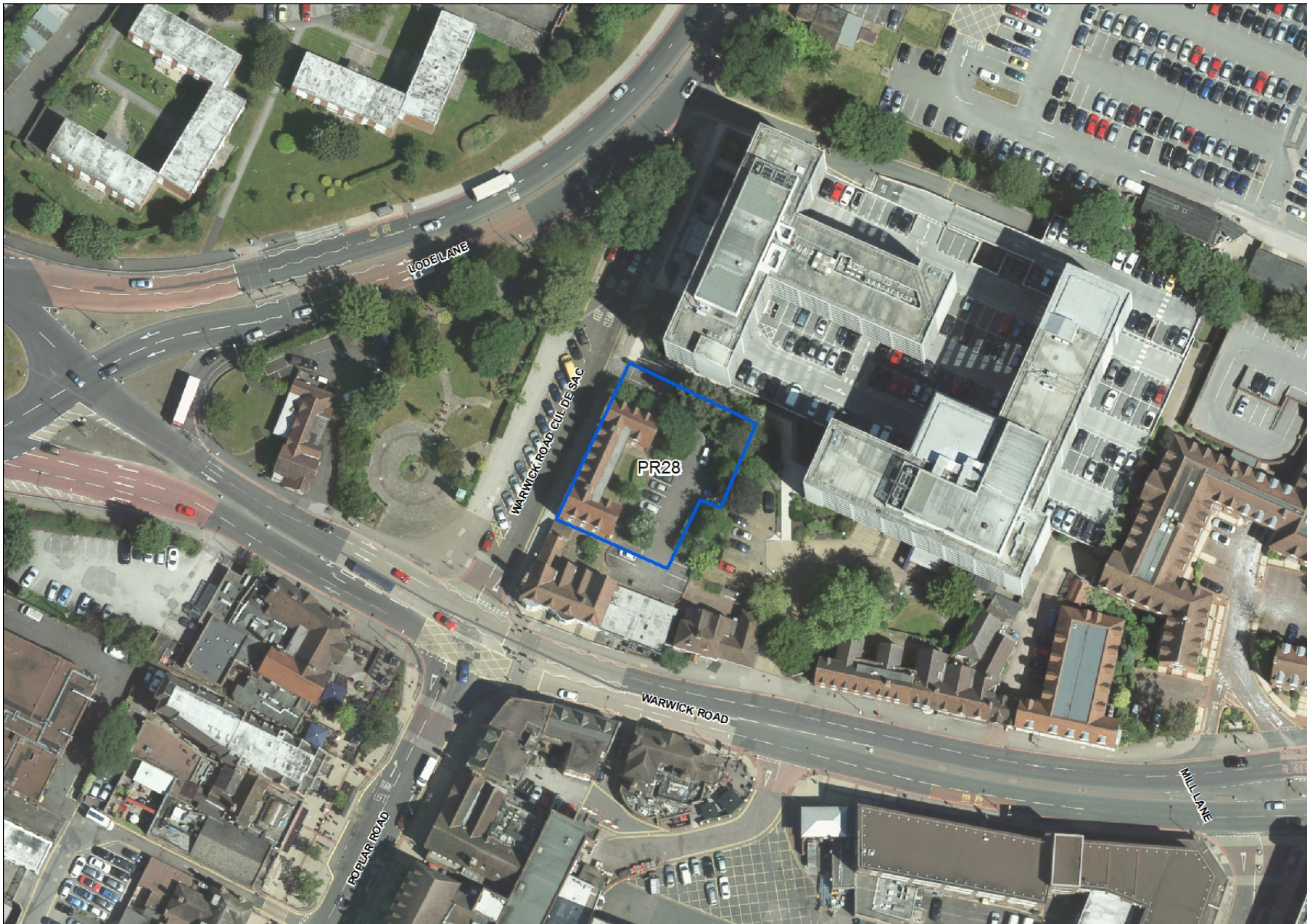
PR28 - Marlborough House, 679 Warwick Road, Solihull B91 3DA
