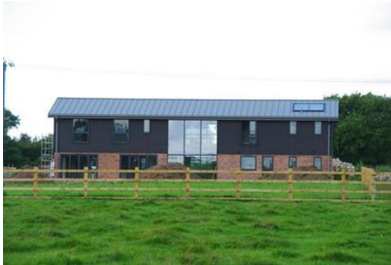
“Framed” barn conversion, Barrett’s Lane Farm
