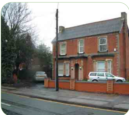
Above: The neighbouring buildings used to establish the typology for the site
