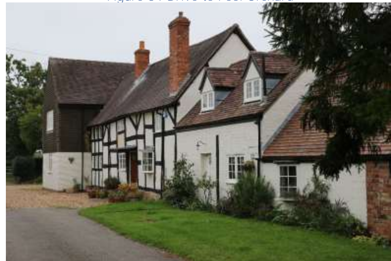
Figure 35 Pool Orchard; north-west elevation with late C20 extension at left
