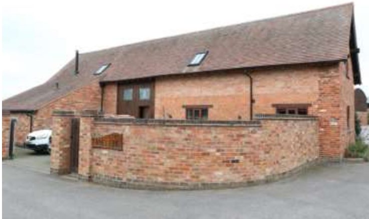
Figure 12 Part of the complex of converted farm buildings at Whitlocks End Farm
