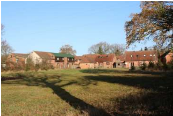
Figure 13 Part of the complex of converted farm buildings at Whitlocks End Farm
