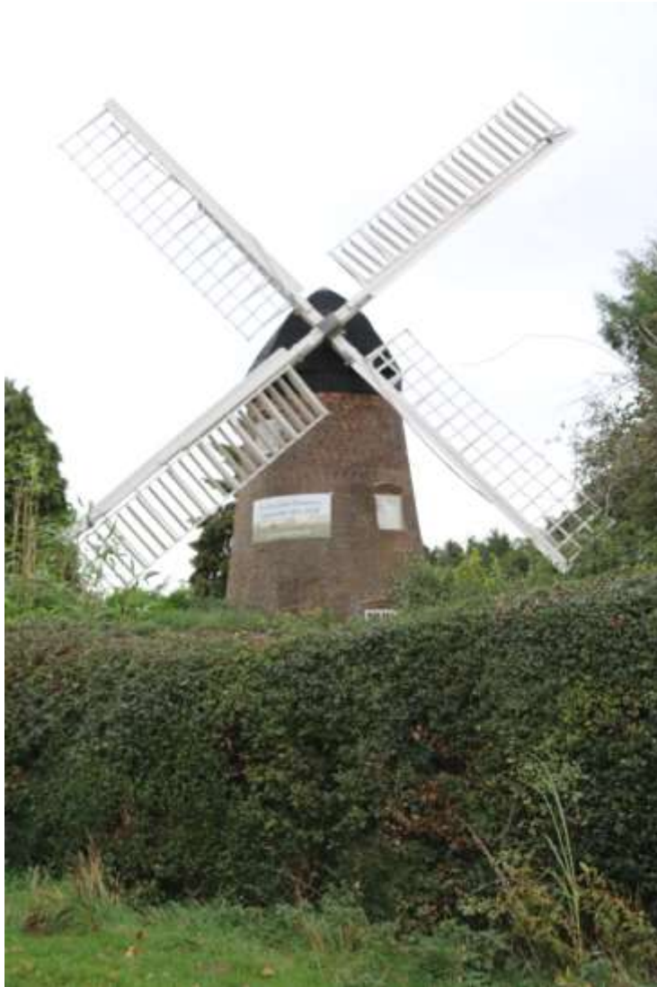
Figure 14 Berkswell Windmill from Windmill Lane adjacent to mill
