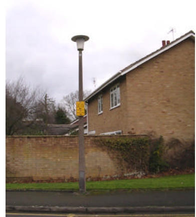
Fig 17: Concrete street light
