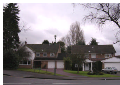
Fig 12: Houses near entrance from Blossomfield Rd
