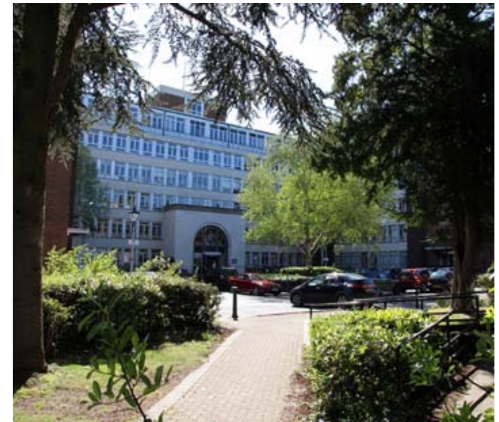
Figure 3.4.5.3 Church Hill House
