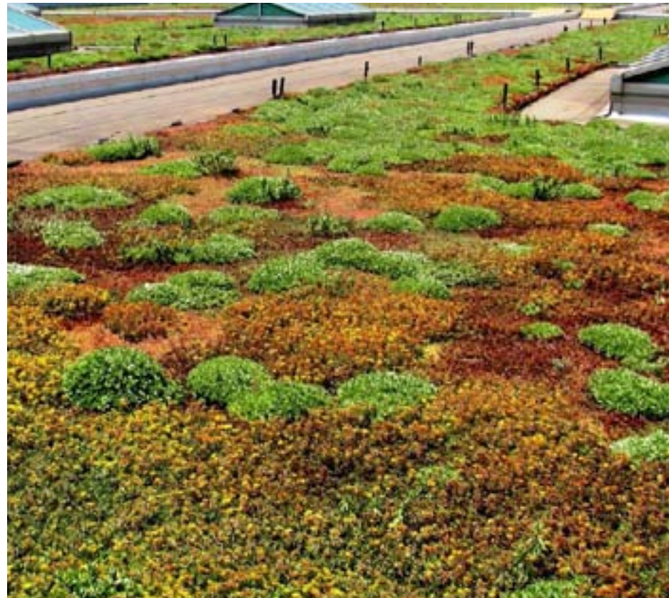
Figure 4.7.10.2 Green roof with sedum planting
