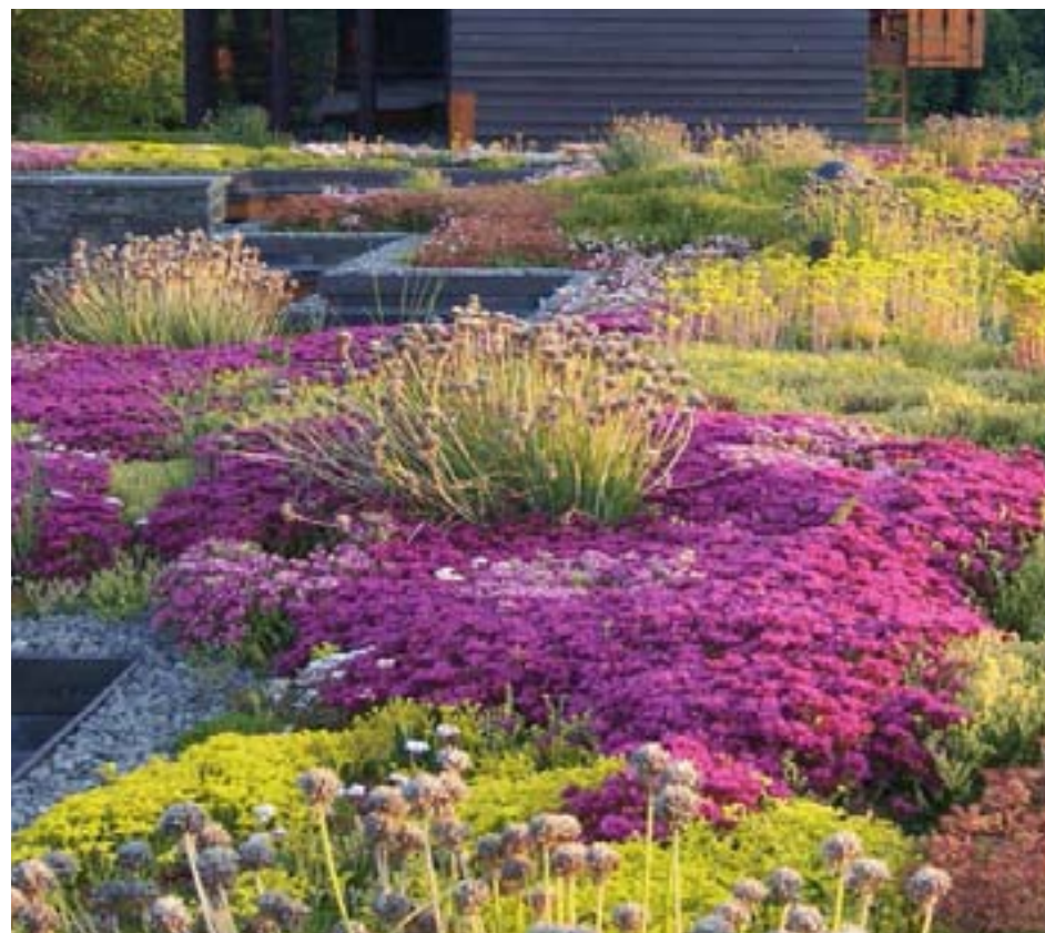
Figure 4.7.10.4 Green roof with hardy shrubs and perennials planting
