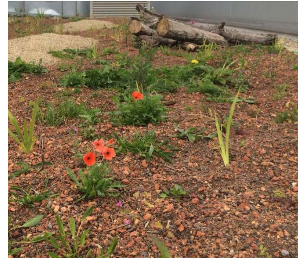
Figure 4.7.10.3 Brown roof example
