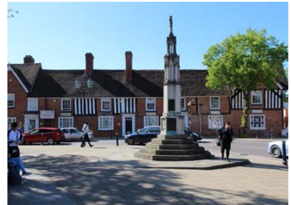
Figure 3.4.3.25 Listed building fronting The Square
