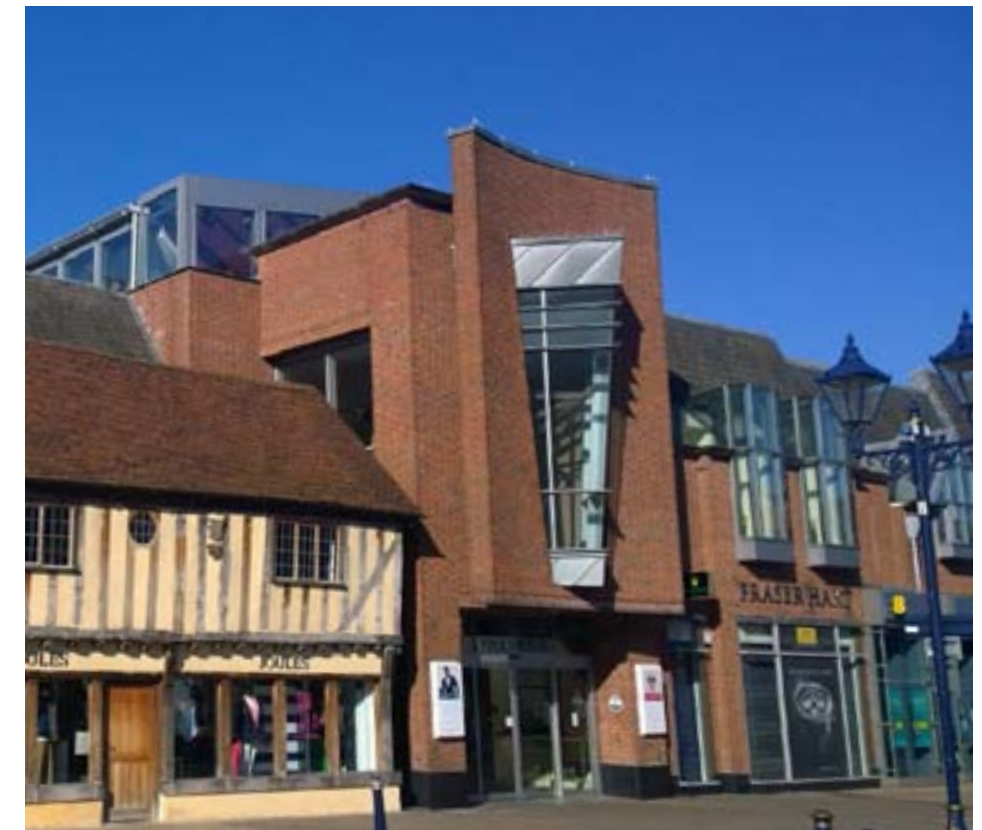
Figure 3.4.3.11 Existing Mill Lane entrance
