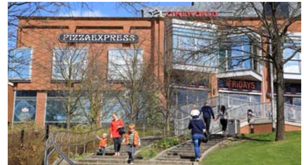
Figure 5.4.1 South west entrance
