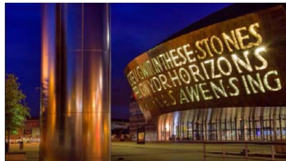
Figure 4.9.7.5 Backlighting to perforated metal screen installation example
