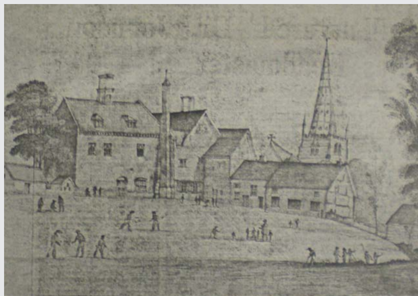
Figure 82: Powell's School 'old Priory', now demolished
