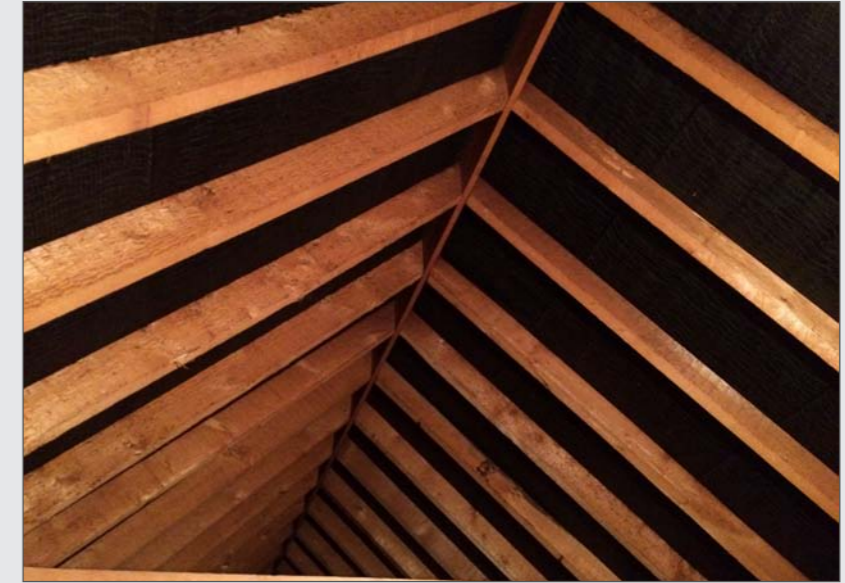
Figure 71: Timber rafters 146 & 148 High Street
