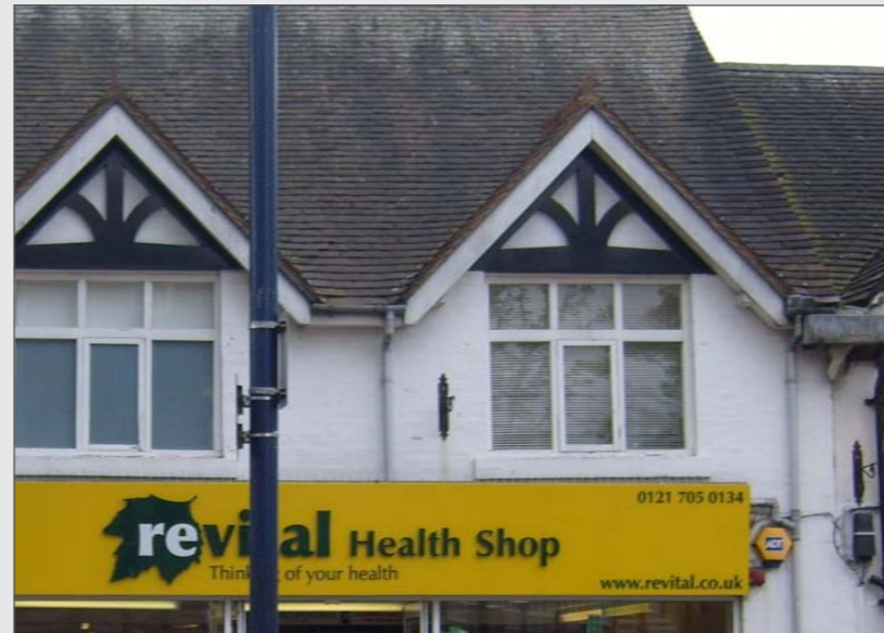
Figure 67: Gabled casement windows to upper storey
