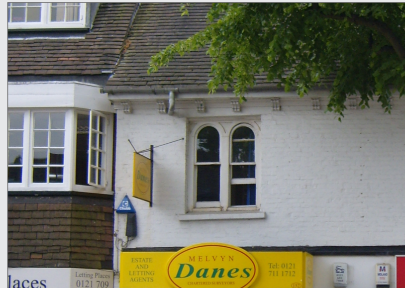
Figure 59: Round headed windows to upper floor
