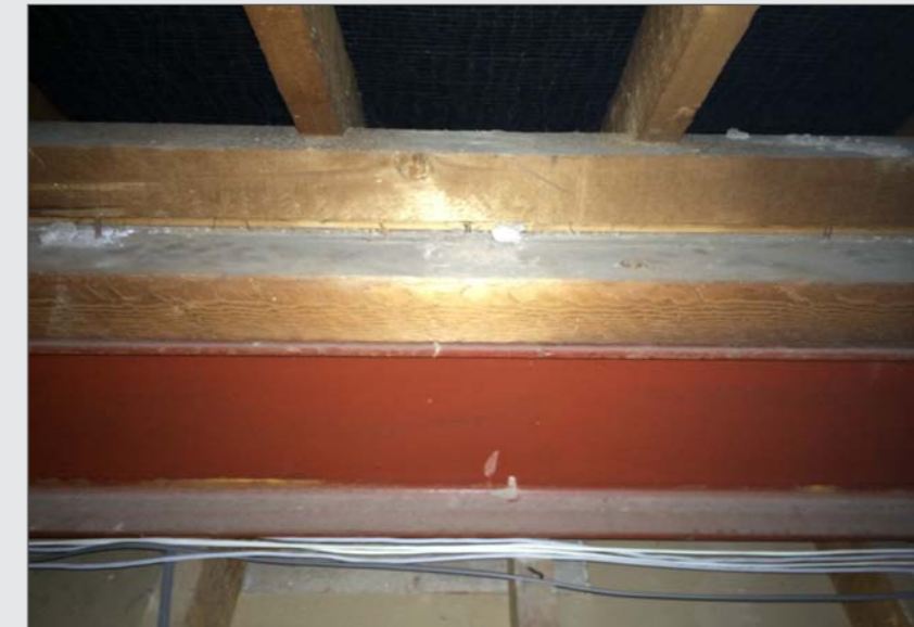
Figure 65: Steel beam over wallplate on front elevation
