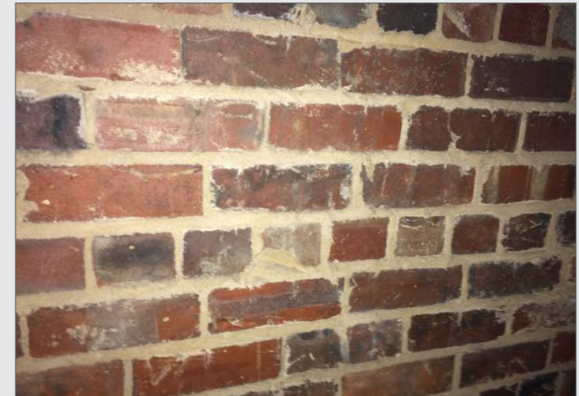
Figure 73: Internal gable wall 146 & 148 High Street
