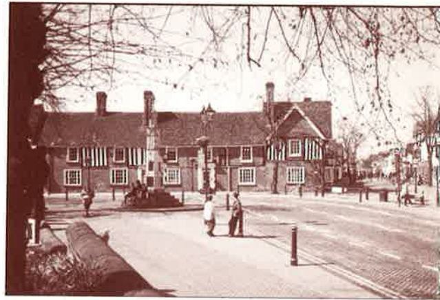
2- 6 The Square and 158 High Street
