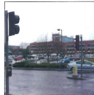
The edges of the centre are dominated by car parking (surface and multi-storey)
