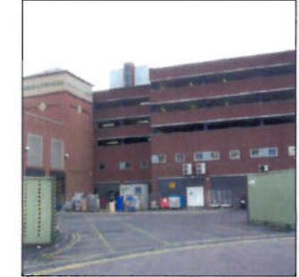
Service Yards and car parks on Warwick Road
