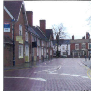
Existing buildings around St. Alphege's
