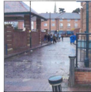
Poor pedestrian link between Morris and Mell Square
