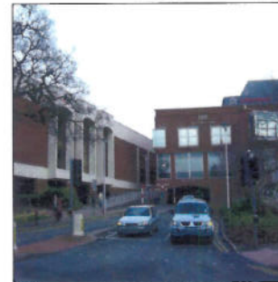
Entrance to underground car park
