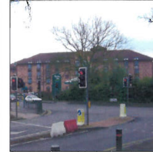
The view of the Holiday Inn from the entrance to Touchwood car park
