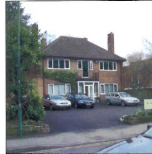
Well designed houses along Hermit Road
