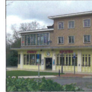
Corner creates a weak landmark at station Road
