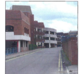
The Multi Storey car park and service road behind the shops on Station Road
