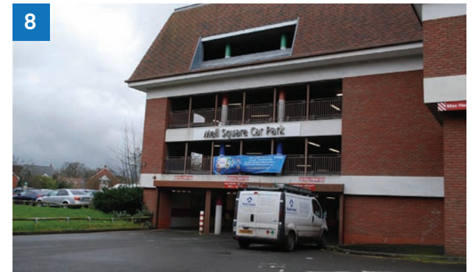
8 Frontage along Warwick Road: Photo shows both multi storey and ground level car parking along Warwick Road. This creates a poor frontage to Warwick Road and a negative pedestrian experience.
