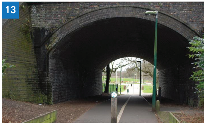
13 Railway underpass connecting Tudor Grange Park and Solihull Town Centre: the underpass can present safety concerns particularly in the evening, due to poor lighting and little overlooking.
