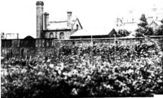
The factory, adjacent to Solihull Lodge.
